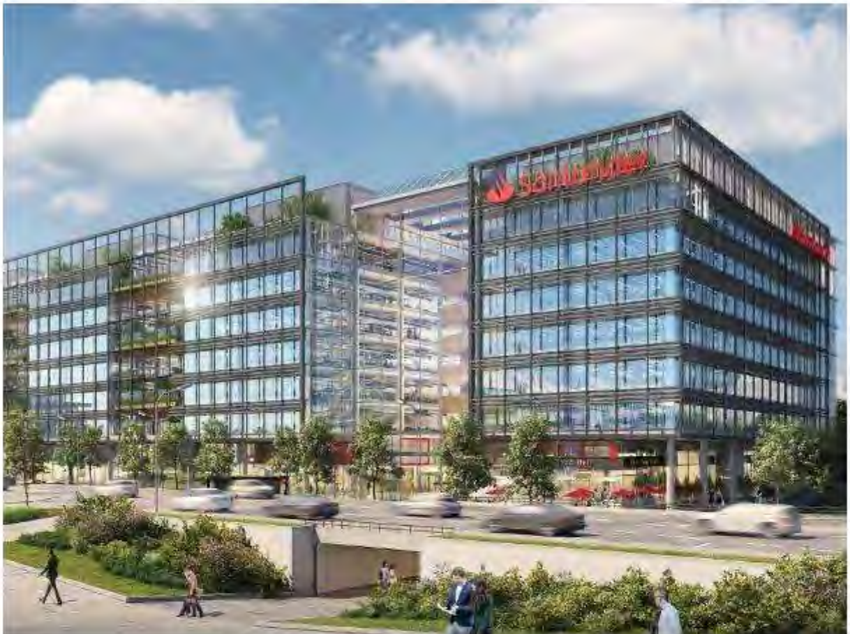
Figure 17: New Santander HQ adjacent to Milton Keynes rail station
