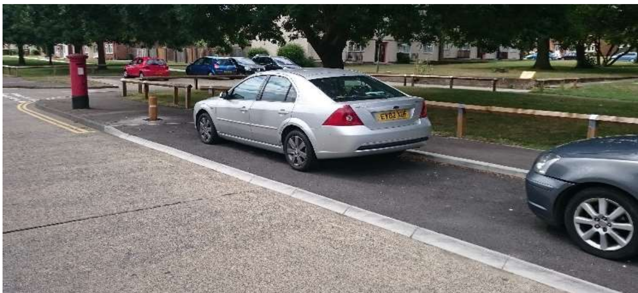
Figure 25 – Example of converted parking lay-by from grass verge
