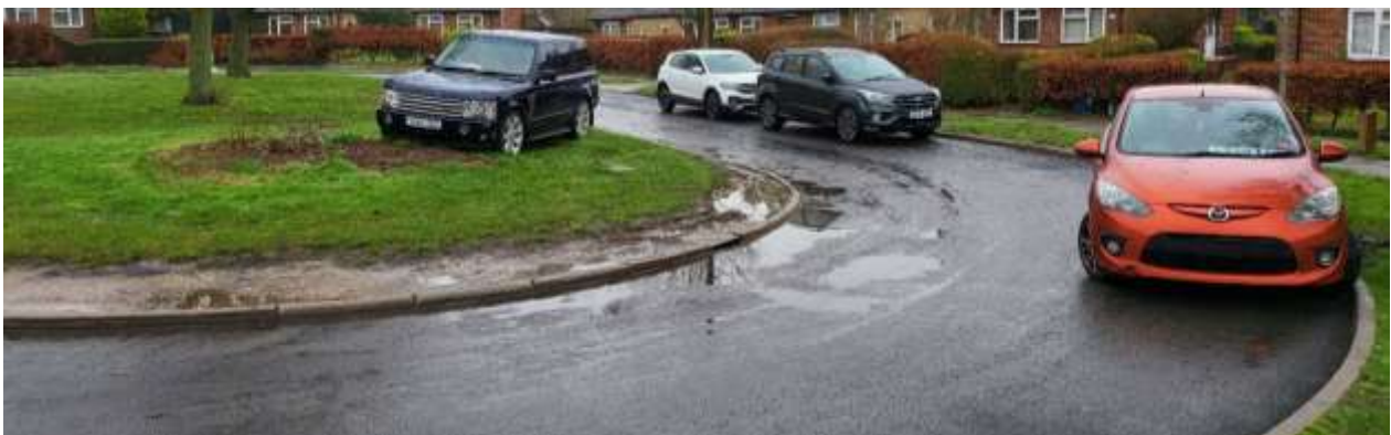
Figure 9 – Examples of verge parking damage along Barclay Crescent, Hawkes Lane, and Ryecroft
