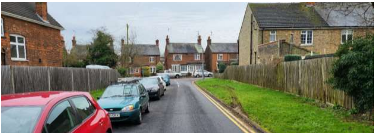
Figure 23 – Example of verge damage that can be resolved through verge protection
