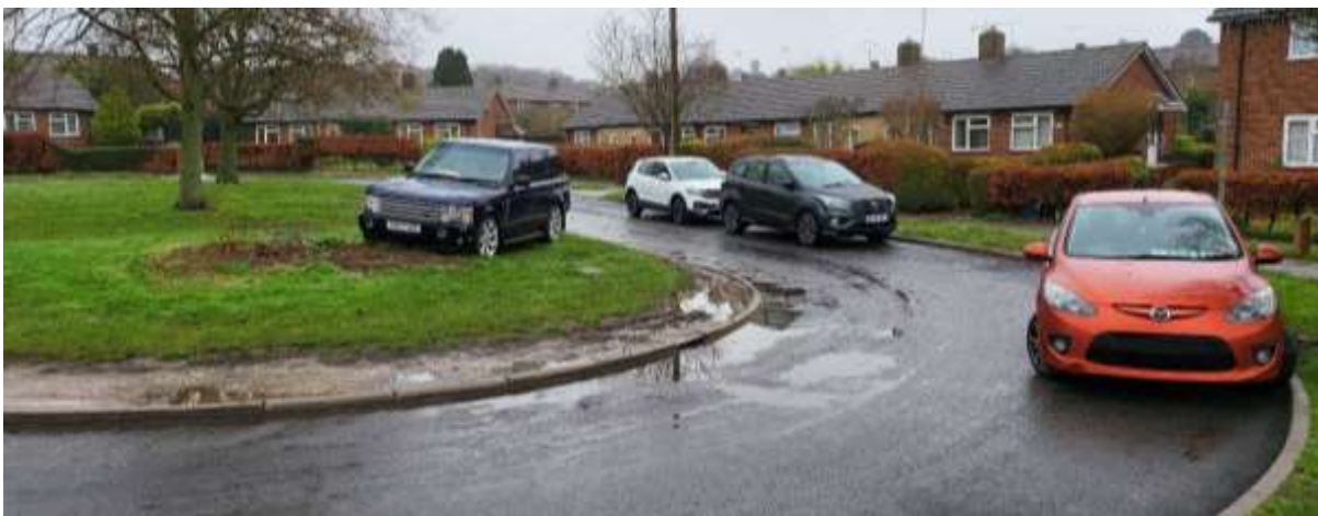
Figure 11 – Example of verge damage caused by parking in Ryecroft;
