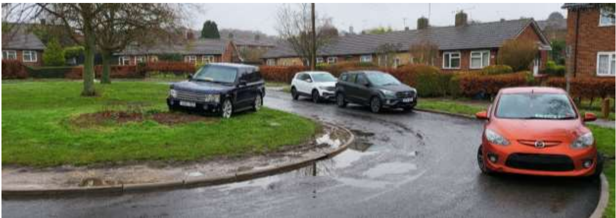
Figure 22 – Example of verge damage that can be resolved through a prohibition order
